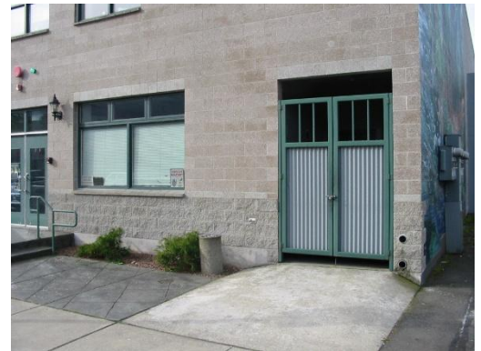
Example of a dumpster enclosure incorporated within the building.
