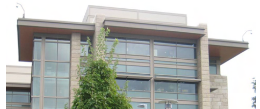
Commercial building using a setback parapet, or "utility penthouse," to screen mechanical equipment.
