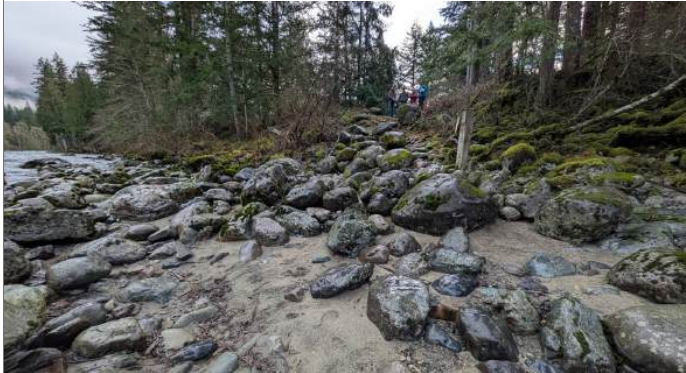
Existing conditions of potential boat launch stairs
