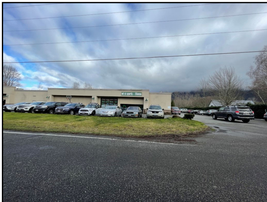
Existing industrial use
