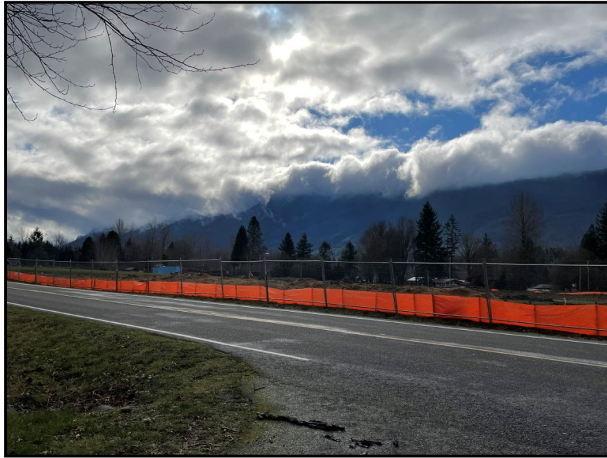
Snoqualmie Valley Athletic Complex project (Phase I under construction)
