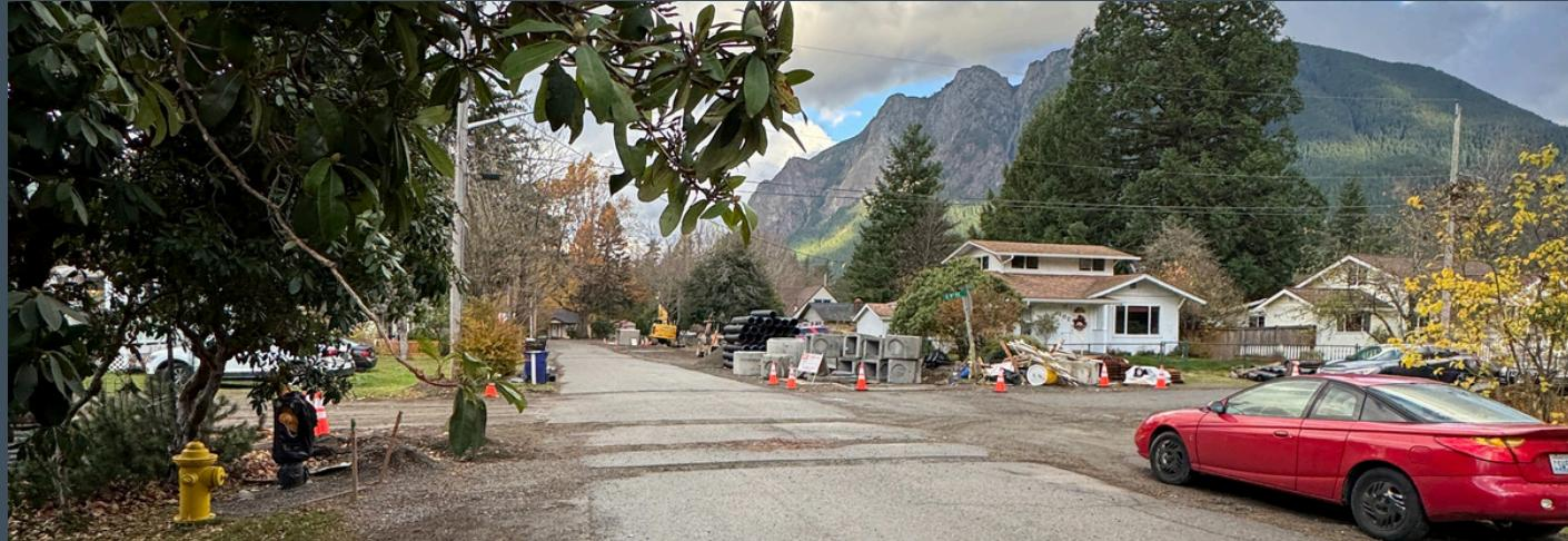
Crews from Ryatt are working in the Old Silver Creek neighborhood: constructing sidewalk, storm drainage and watermain for 5<sup>th</sup> St, 6<sup>th</sup> St and Main Ave. They're swapping water services over to the new water main the week of November 10, with water main work wrapping up by the end of November. They continue in working to install stormwater infrastructure along Main Ave and will soon be installing storm drains down 6<sup>th</sup> St.
