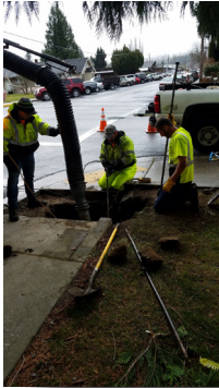
Public Works Team replacing broken fire hydrant
